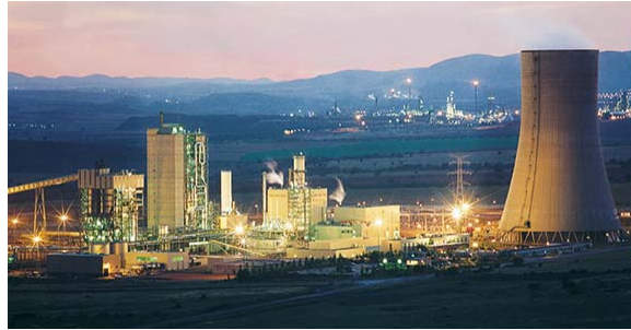
IGCC plant at Puertollano, Spain
